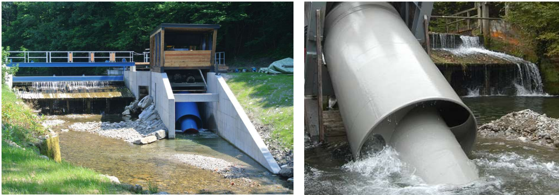
Figuur 13: Hydroconnect vislift (bron: www.hydroconnect.at )
